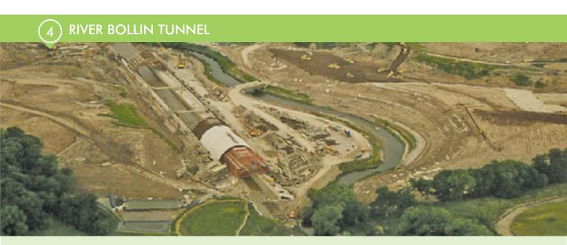
The tunnel was created to carry Runway 2 across the River Bollin and at 240m long, 18m high and 24m wide, it is in itself an impressive piece of engineering.
